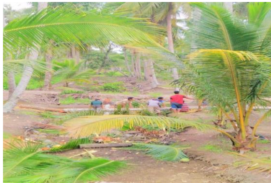
Figure 2 Work Devotion Cleaning ditch
