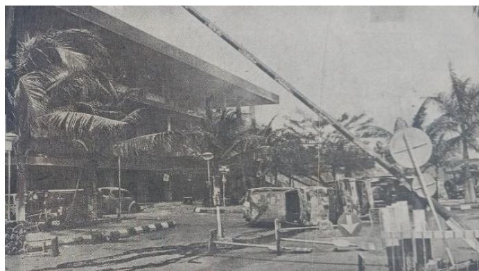
Figure 2. The Senen Project after being set on fire by demonstrators.
