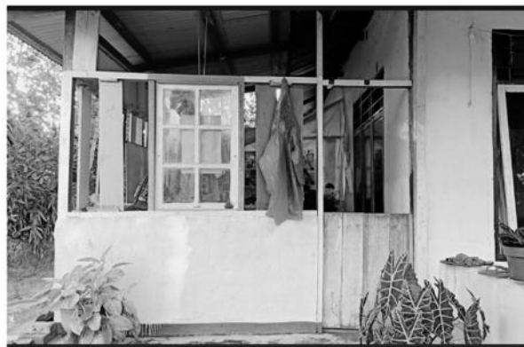
Figure 2. The TBM Keik Tsinagi occupies an ancillary room constructed adjacent to the main residence
